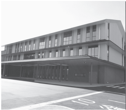
御所市防災交流館 Gose City Disaster Prevention and Community Center Mimoro
